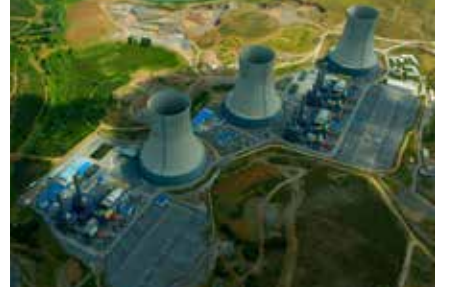
Enka Power Plant – Erbil – Süleymaniye
